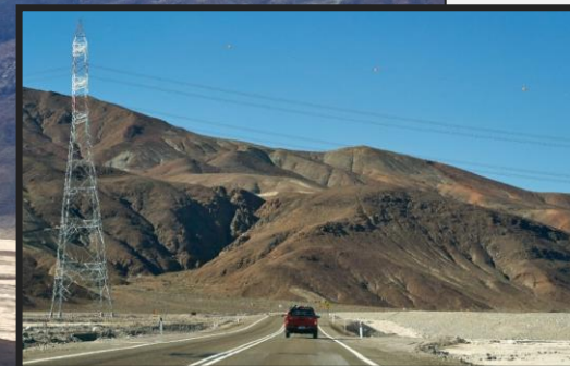
Paved highway & 2 powerlines cross the property
